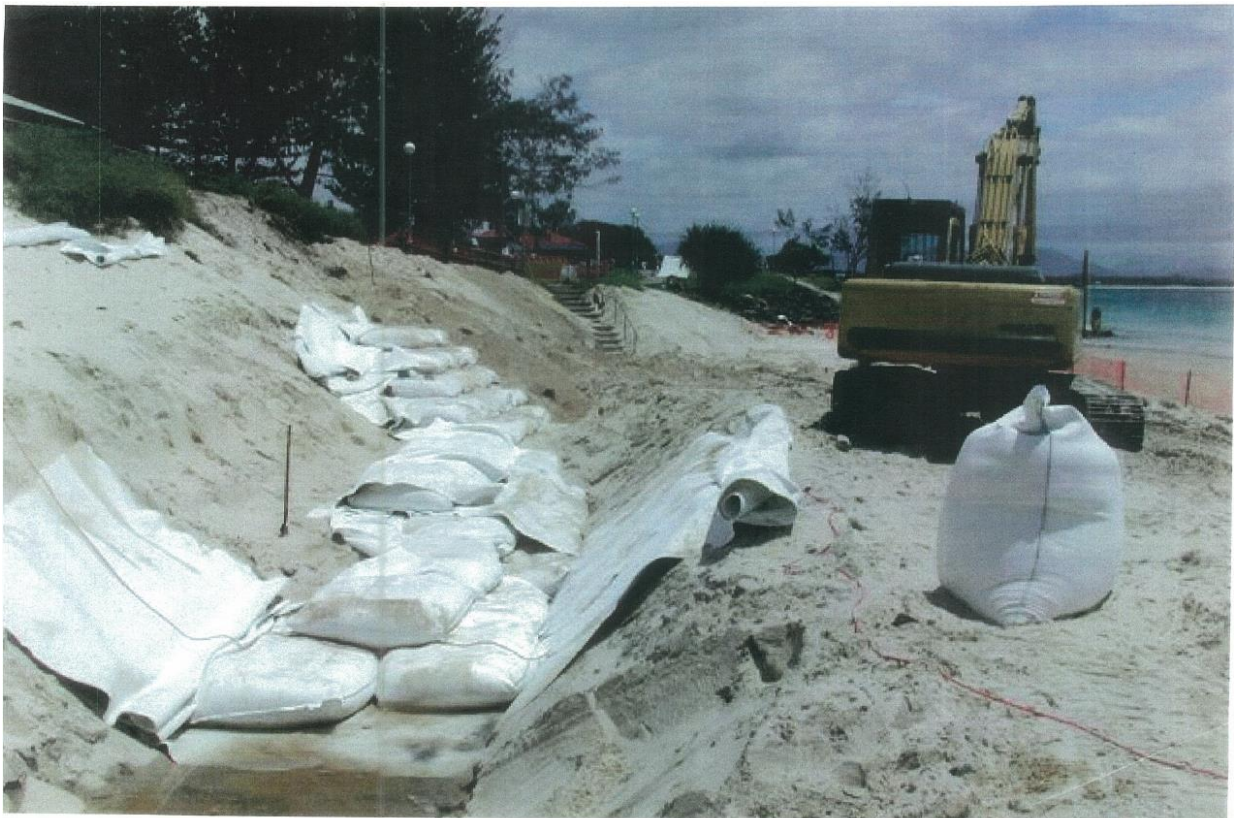
Figure 5: Construction of geobags fronting Byron Bay SLSC c2001 (Source: Byron Shire Council)
